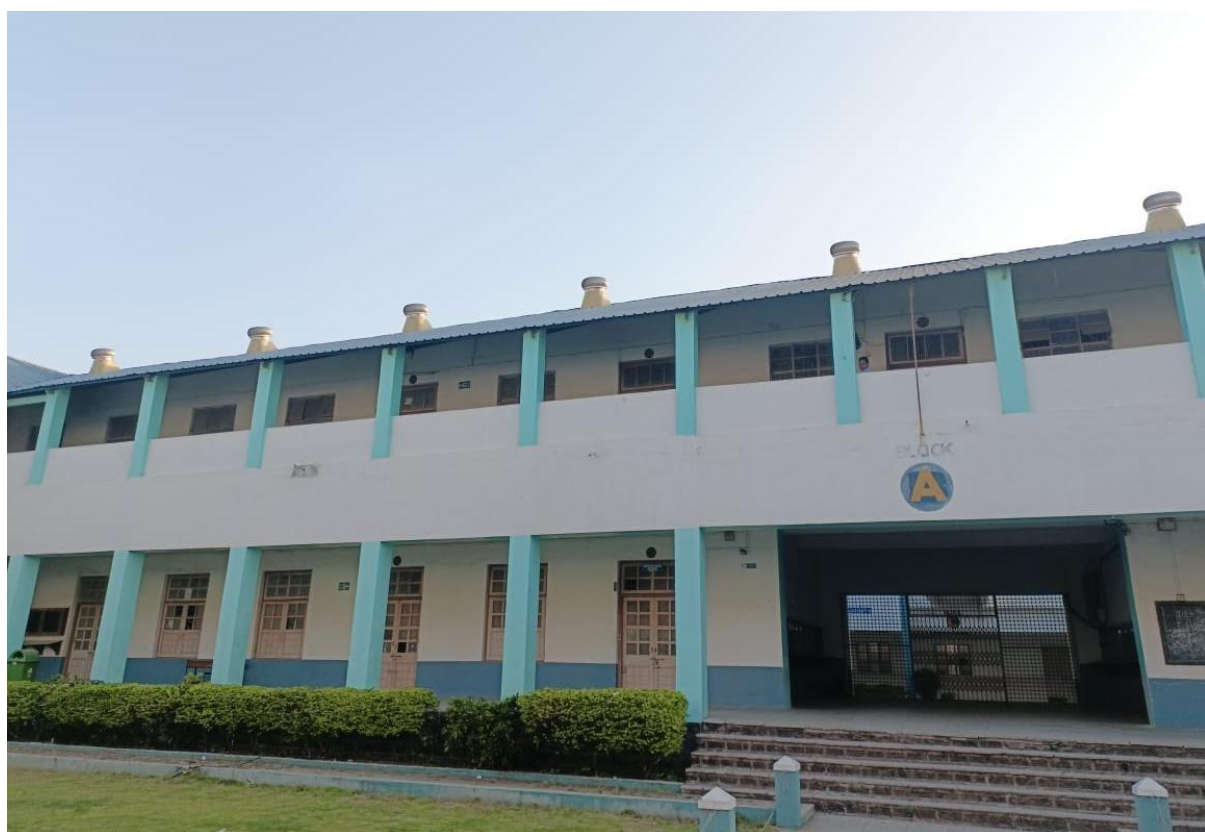
Turbo Ventilators in the campus building
